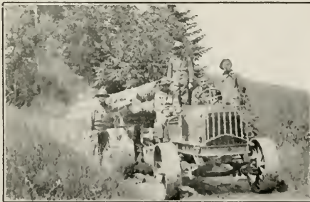
46 CO. LOGGING OPERATIONS.
