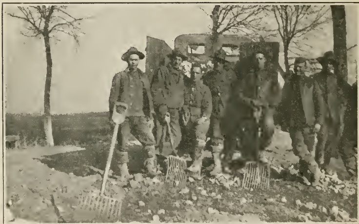
ROAD RECONSTRUCTION A detail of the Forty-Third Engineers
