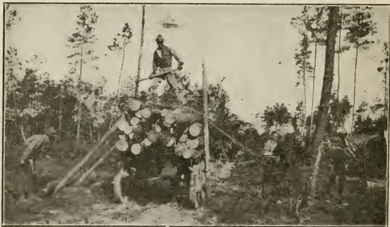
LOADING LOG WAGON WITH CROSS HAUL
