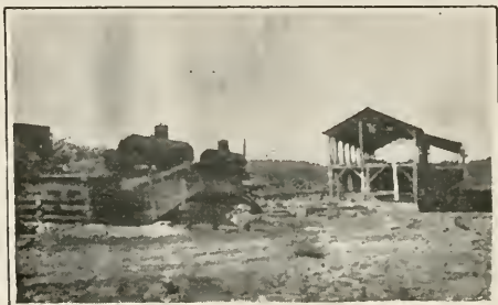
LAMARCHE MILL UNDER CONSTRUCTION.
